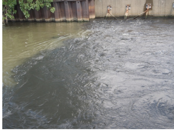
Figure 7. Rouge River DWSD Outfall #050, 8-9-11.
